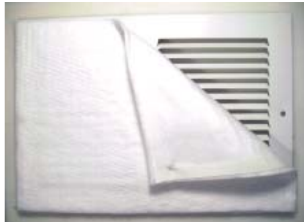
Medical Filter Installed on Return Vent
